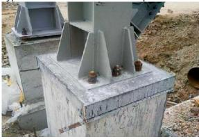
The compressive strength of the grout must exceed 50 N/mm<sup>2</sup> at 7 days and 60 N/mm<sup>2</sup> at 28 days.
